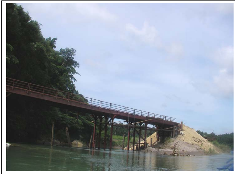
Temporary bridge built to facilitate construction of the dam
