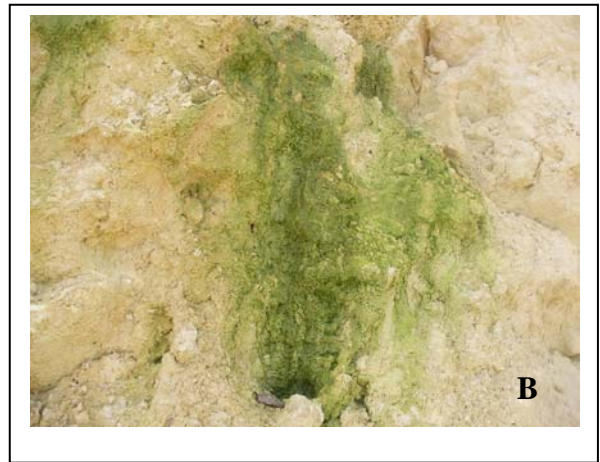
A and B: Calcarenite limestone showing pores where water comes out and algae tends to grow
